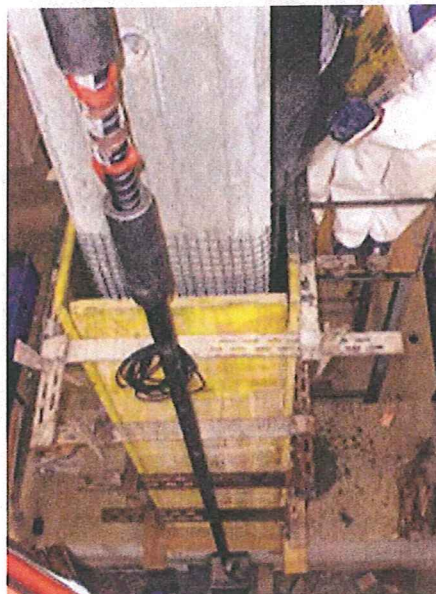
Fig. 5: High-performance jacket casting
